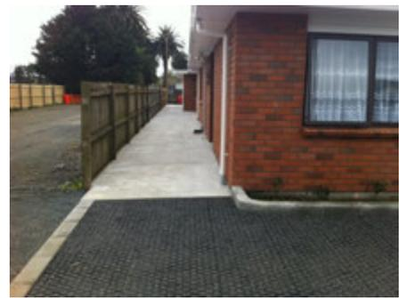
**3** A decorative river pebble 5 - 10mm (discrete) was used for the filling and capping the **JakMat Geocell**.
